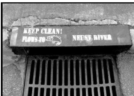
Figure 1. This stenciled storm drain educates the public about where stormwater flows. Photo courtesy of the City of Kinston.
